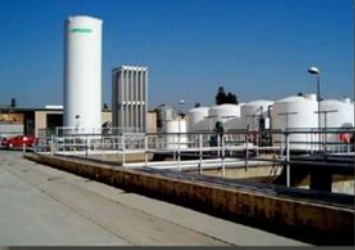
The ET Process plant in Fresno, CA, owned by Cottonwood Creek Biosystems, takes in tankered grease and food processing wastes and generates single cell protein and dischargeable water.
